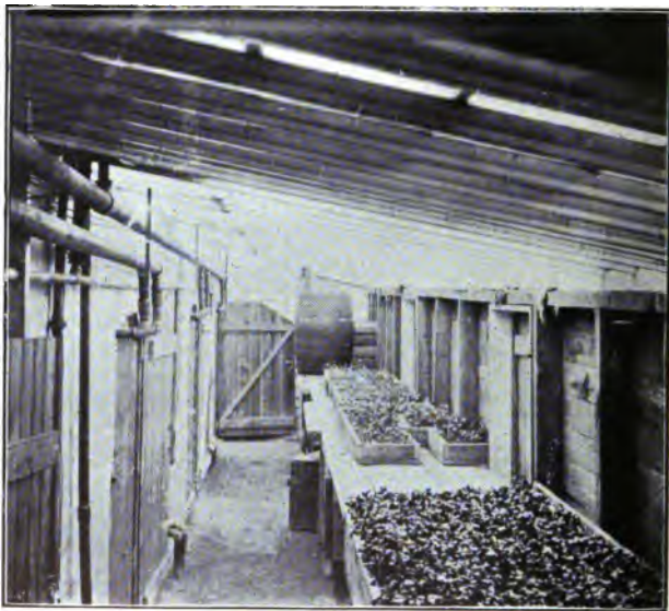
11.—Interior of shed shown in 10. Propagating bench on the right, supply pipes (two inch) on the left, shed eight feet wide.
